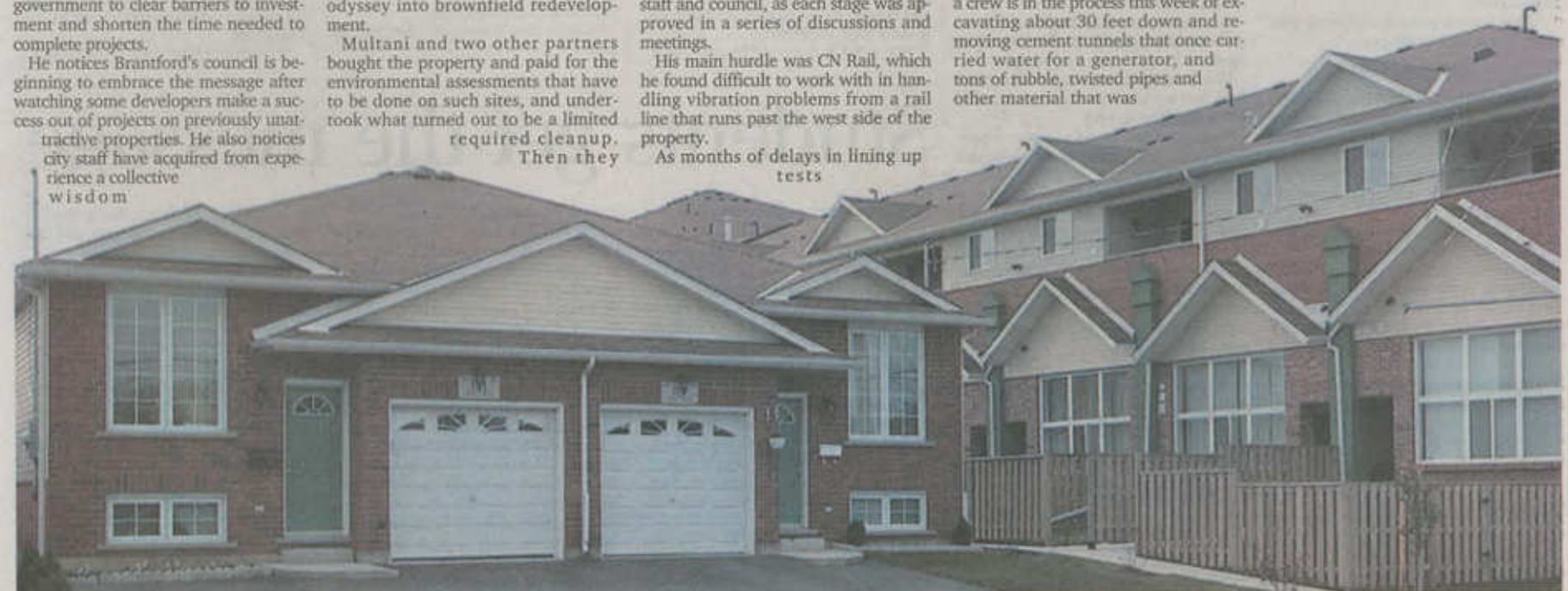
The Multani development on Grey Street includes semi-detached houses and a large condominium apartment complex.
